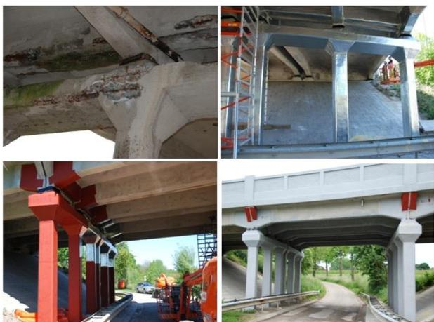
**Effectiveness:** ZLA eliminates corrosion by operating as a galvanic anode
