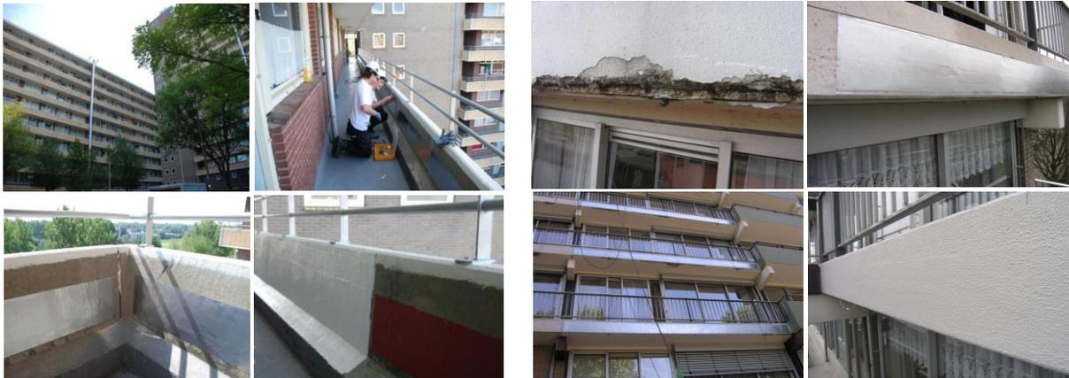
ZLA is provided in rolls (250 mm wide by 25 meters long). After application ZLA should be finished with an approved cementitious based coating of the specified texture and colour, ensuring edges and seams are properly over coated to avoid moisture ingress. System monitoring can be performed according to the standard ISO 12696.
