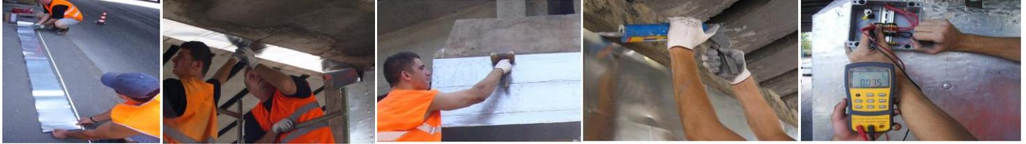
After cutting the ZLA into the appropriate length can be applied onto a cleaned concrete surface by hand application. Old concrete surfaces must be structurally sound with any unsound areas being repaired prior to the installation of ZLA. Laitance and other surface contaminants also need to be removed.
